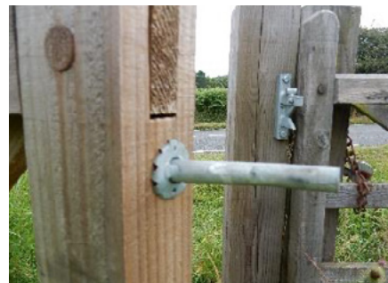
A protruding sharp-ended metal bar such as this can easily injure a horse or catch on a saddle or rider's leg when trying to negotiate a gate. A rubber stop fitted across the end or triangular closed end bar reduces the risk.
